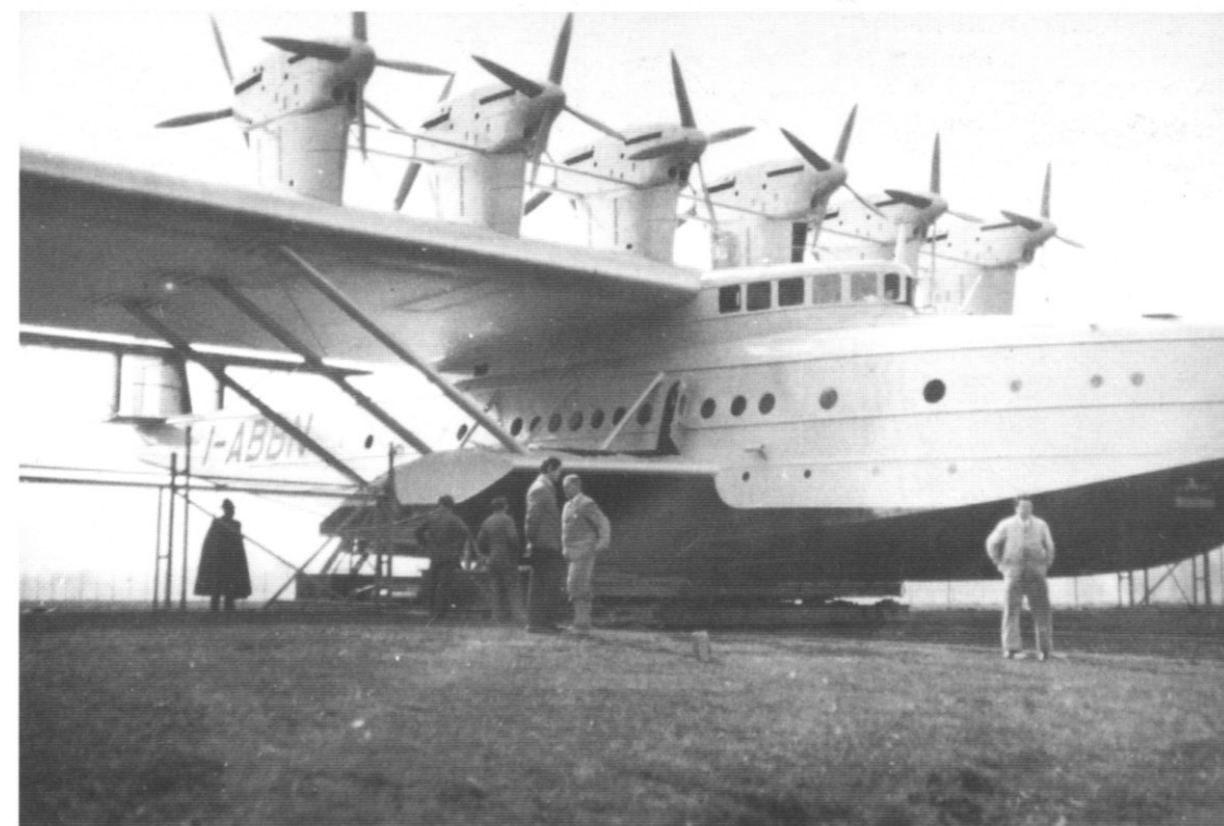
Another version of the Do X coded I-ABBN with Fiat engines. (Dornier GmbH)
