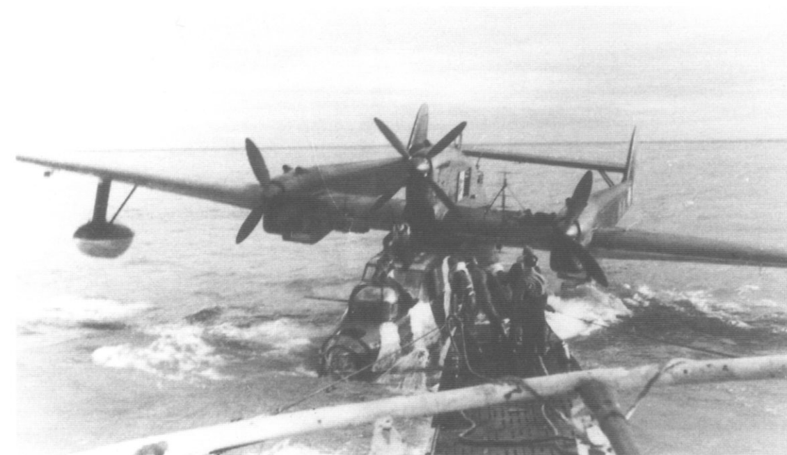
Arctic rendezvous. An unidentified U-boat meets up with a FuG 200 'Hohentwiel' radar equipped BV 138 C of 2/130 for refuelling near the Arctic convoy routes; the second photo shows the same seaplane on its return to Norway, 1943-44. (Drepper)
